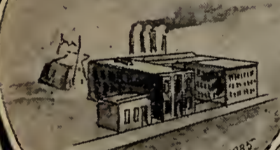
HIGHLAND PLANT ESTABLISHED IN 1885.
